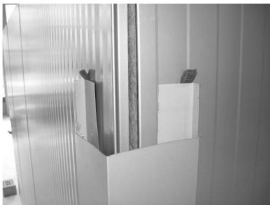
The more elegant corner detail using a concealed support angle. A Type 4 sealing tape must be installed between the panel surface and the support angle. The fastening brackets can be fitted using self-drilling screws. The corner cladding itself is fastened to the sides of the support angles using coated aluminium rivets with a stainless steel mandrel.
